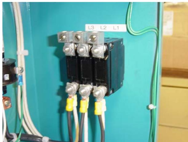
Figure 1.1 Internal view of the main breaker for connecting incoming power.
